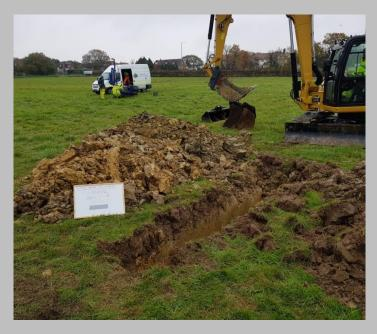
Trial pitting is usually undertaken using a tracked 360° excavator or JCB 3CX backhoe excavator. Concrete breaker attachments are available for sites with hardstanding.
